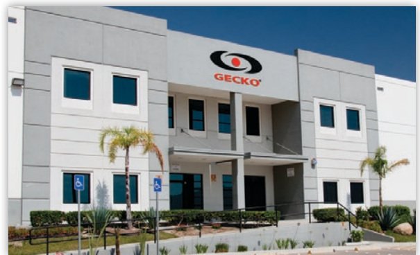
Palmera plant, Tijuana, Mexico
